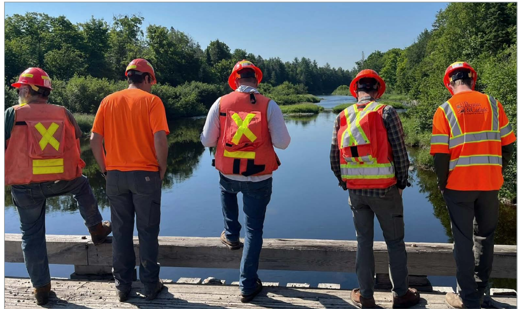
A group of P&C foresters inspect a bridge for integrity during an internal audit.
