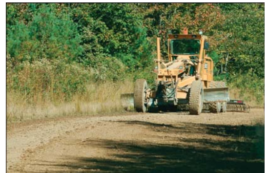
A P&C grader works overtime to ensure our haul roads are in good operating condition.
